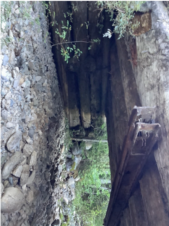
Right Bank Abutment when facing downstream
