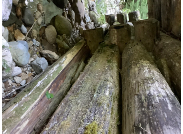
Left Bank Abutment when facing downstream
